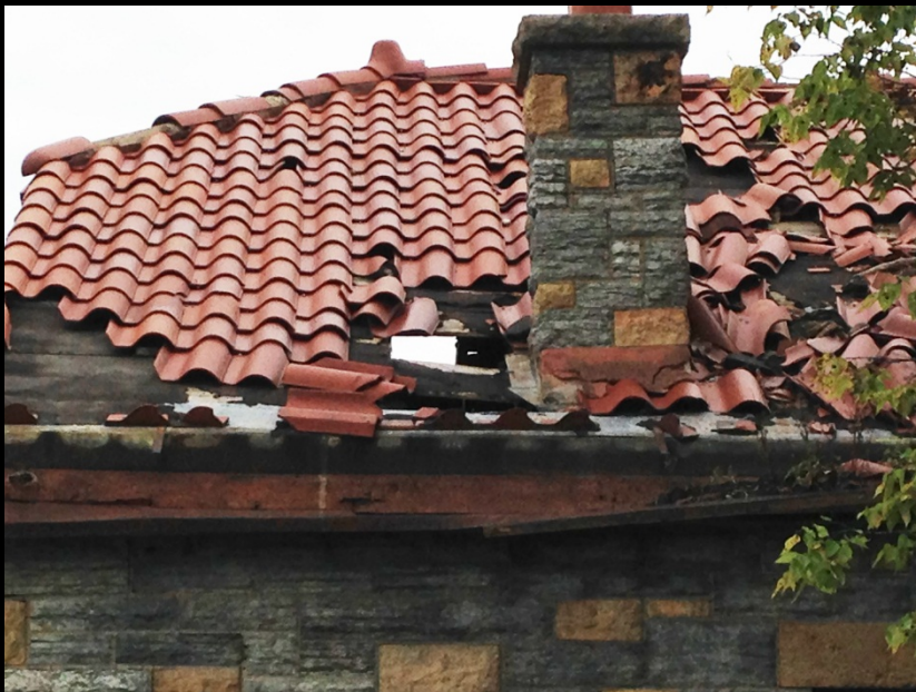
Highland Pool House –Fall 2014
